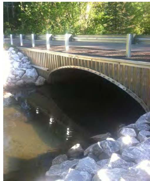
Fig. 3.2.7. Improved Putnam Road Bridge
