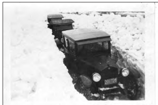
Fig. 3.5.2. Opening Mohawk Trail in Florida MA with Shovels 1926
