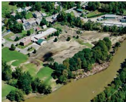
Right: Sediment deposition due to flood waters in floodplain area
